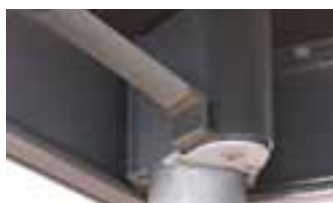
Corner brackets have a cam locking system
